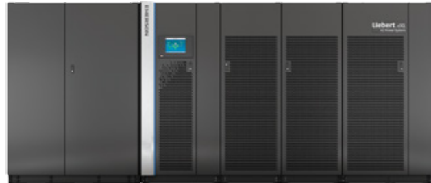
Top Terminal Battery Cabinet
